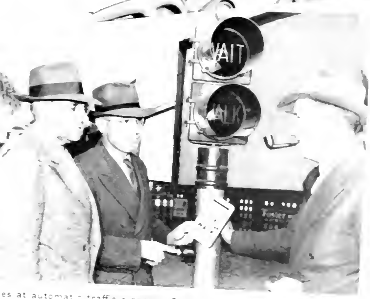
es at automatic traffic signal in San Diego. Top left—Electric brain that receives messages from magnetic traffic detectors and operates signals. Top right—Pedestrians on safety island awaiting effect of push button signal. Center—Market and Pacific intersection. Bottom left—Pedestrian "Wait-Walk" signal. Bottom right—Left turn signal and magnetic detector of buried pavement
